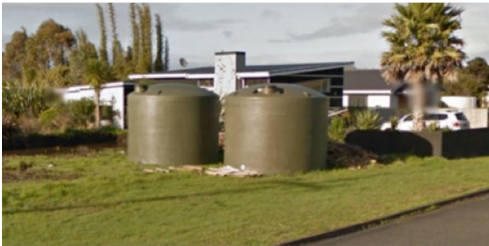
ABOVE FIG. 3-3-4: Private rainwater tanks
