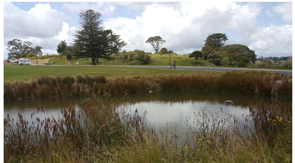
ABOVE FIG. 3-3-3: Stormwater pond in Mangawhai
